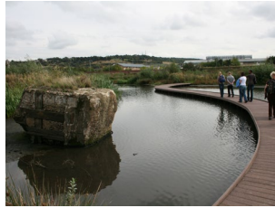
Detention wetland: former steel works Tom Wild, VALUE project
