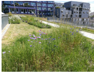
Green roof, Paris. Regreen Project. Image: ARB idF
