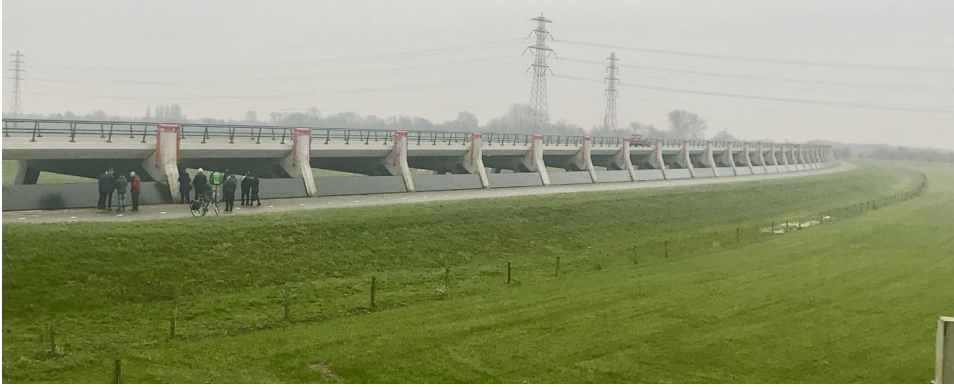
Figure 22. Creation of an additional space controlled by portable flood gates that sit under the road and within the flood plain in the IJssel region in the Netherlands (H2020 RECONNECT project demonstration site). This site is part of the “Room for the River” programme. It aims to provide flood protection, enhance the landscape and improve environmental conditions in the areas surrounding the Netherlands’ rivers. (Photo: Zoran Vojinovic)
