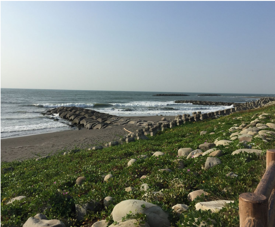
Figure 26. Coastal flood risk reduction with hybrid measures (i.e., combination of hard engineering and Ecosystem-based approaches) in Taiwan, FP7 PEARL project. (Photo: Zoran Vojinovic)
