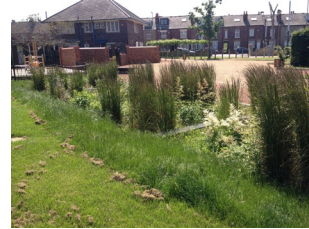
Rain garden - detention, Sheffield Image: Tom Wild
